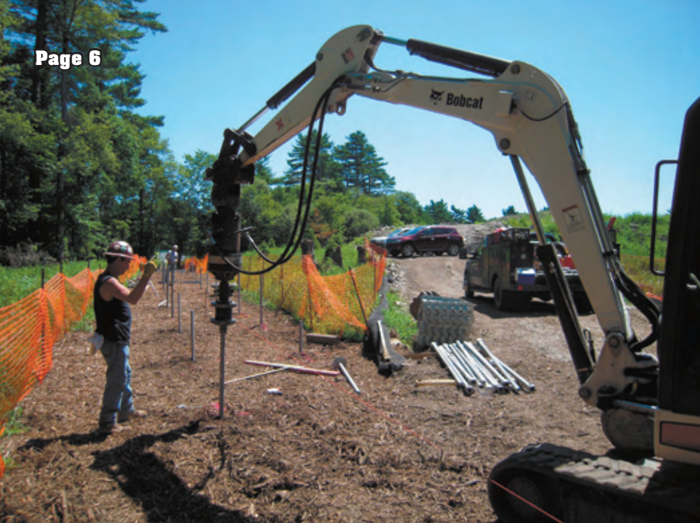
Readings of torque indicator in line with helical pile and rotary drive motor are correlated with empirical charts to determine load-bearing capacity of pile.
