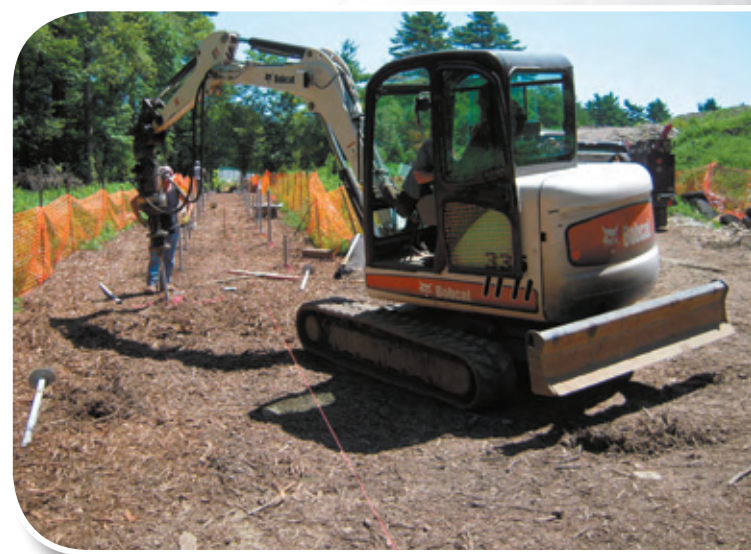
Solid Earth Technologies uses a Bobcat 335 Excavator to install Chance helical piles for boardwalk being built by I.W. Harding Construction in Norwell, Mass.
