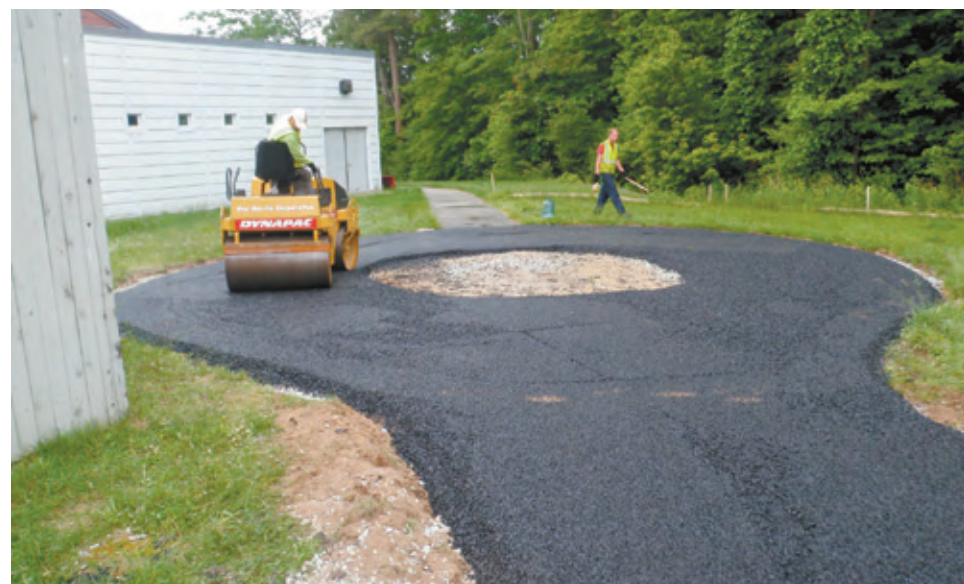
Martin Corporation's DYNAPAC roller compacts porous pavement, which allows water to pass through to an underlying stone recharge bed and into the soil.
