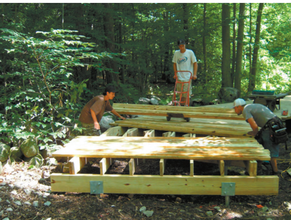
When narrow ROW and other conditions prevented large equipment access, workers used handcarts to bring in building materials for the boardwalk.
